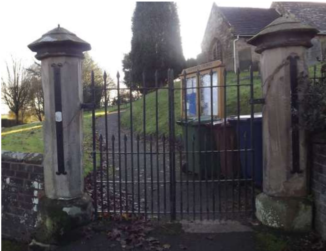
Figure 63 Wrought iron gates at All Saint's Church
