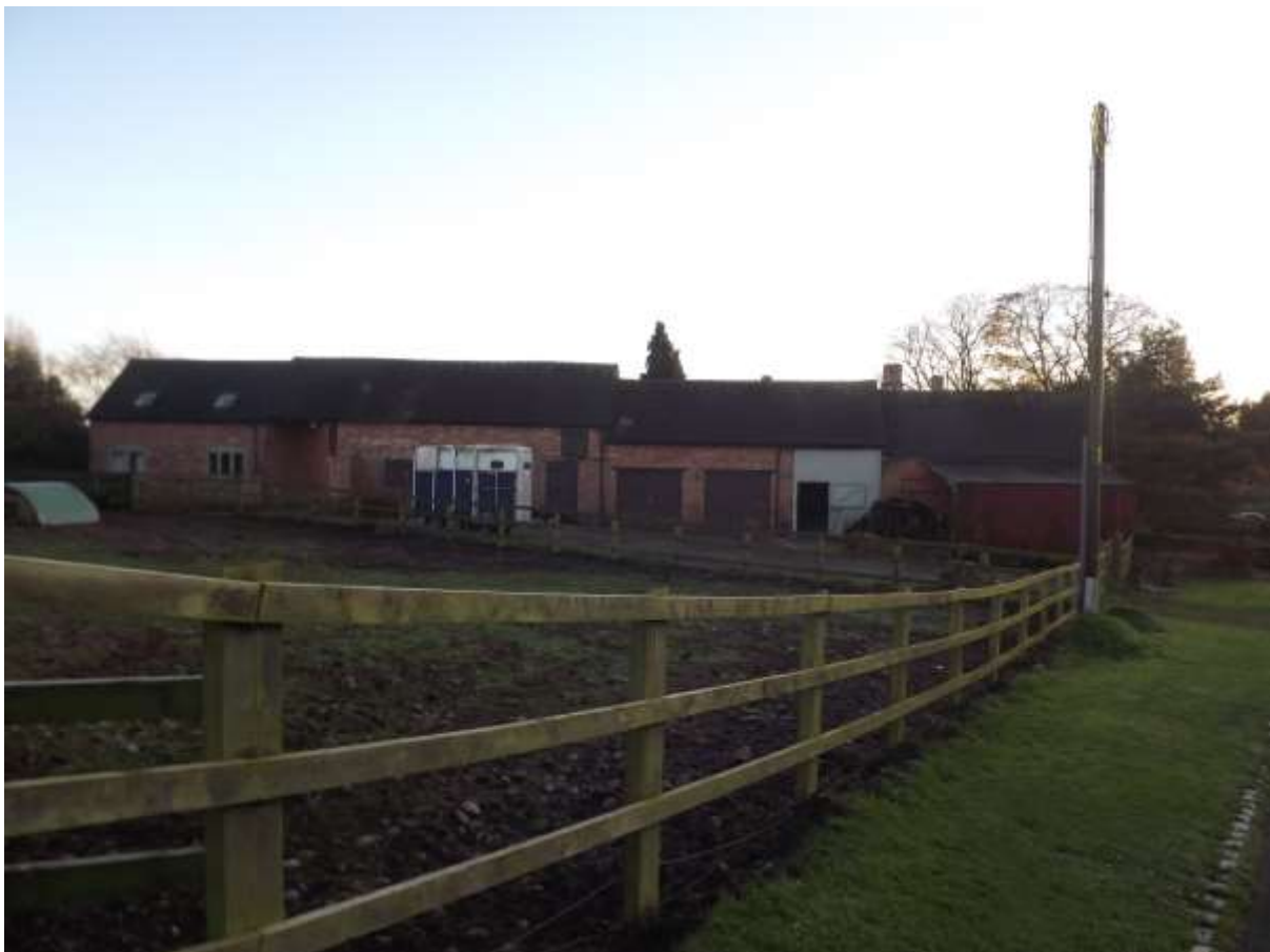
Figure 34 Agricultural buildings to Riverside Farm
