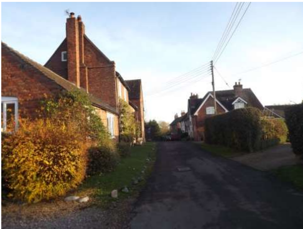
Figure 12 Double stacked external chimney to the Old School House
