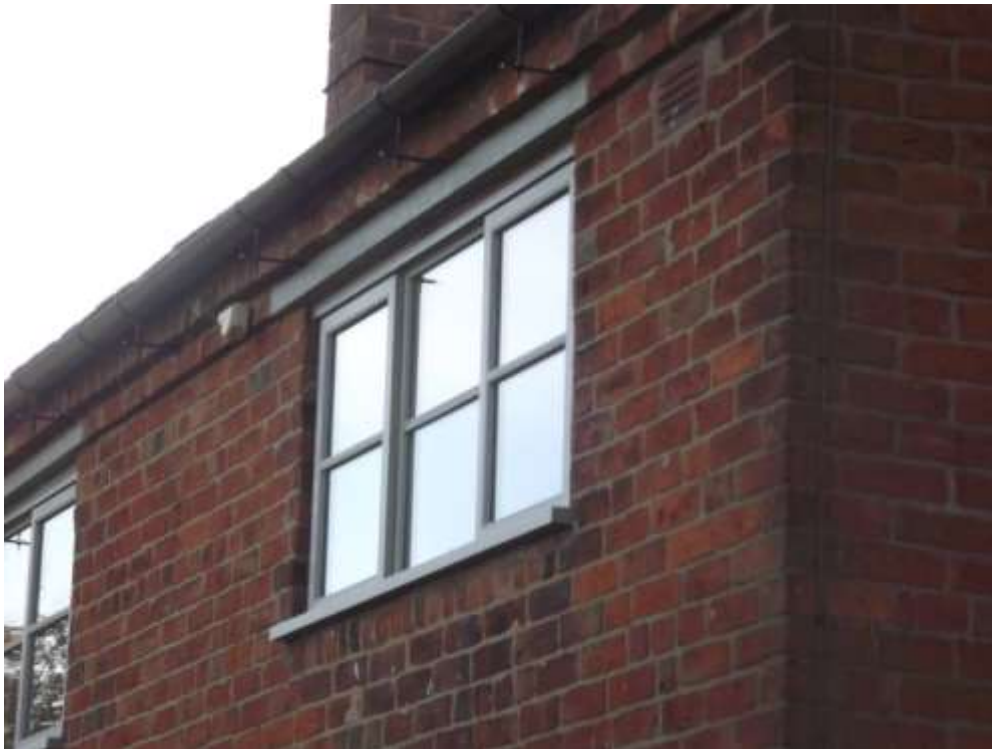
Figure 16 Replacement casement window to Drumble Cottage
