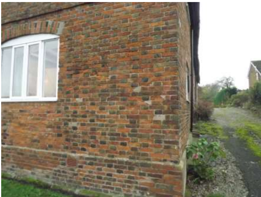
Figure 19 Brickwork to the Old School House
