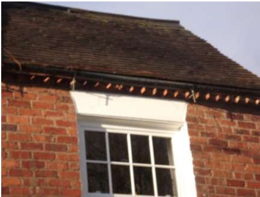
Figure 18 Dentilation at eaves to Croft House
