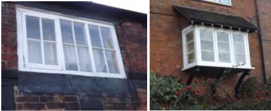
Figure 13 Historic timber pegged window frame and glass at Park Cottages and box style projecting casement window to Old Mill Farmhouse
