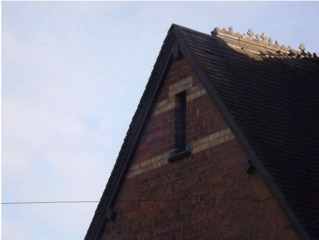
Figure 20 Decorative ridge tiles and slit vent to village hall
