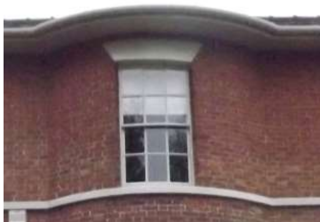
Figure 14 Unusual sash window set in a bow at The Mount
