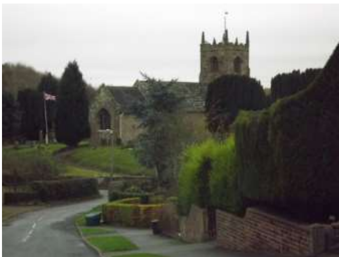
Figure 44 View of All Saint's Church from The Green
