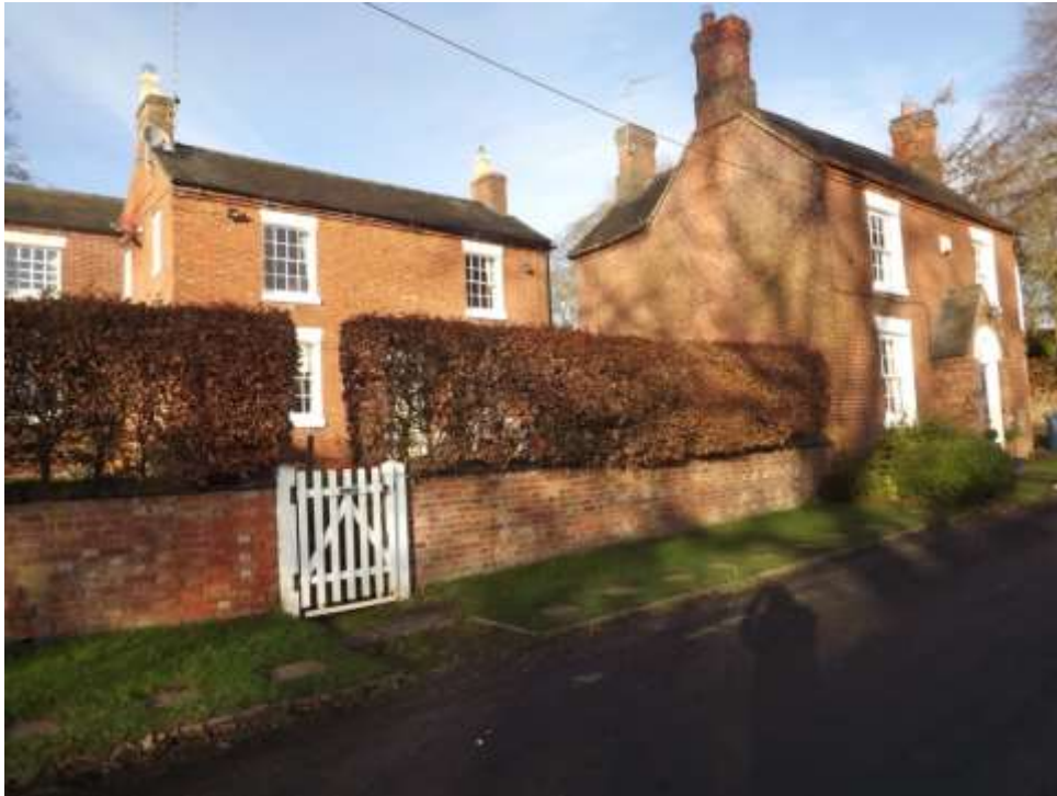
Figure 11 Regular spaced chimneys in gable wall
