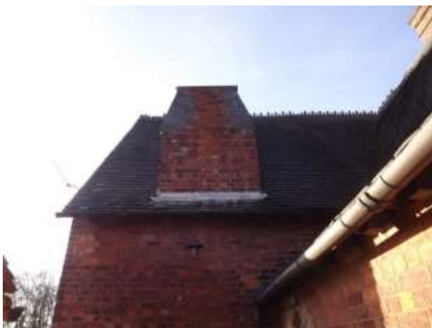
Figure 10 polychromatic brick chimney to the village hall
