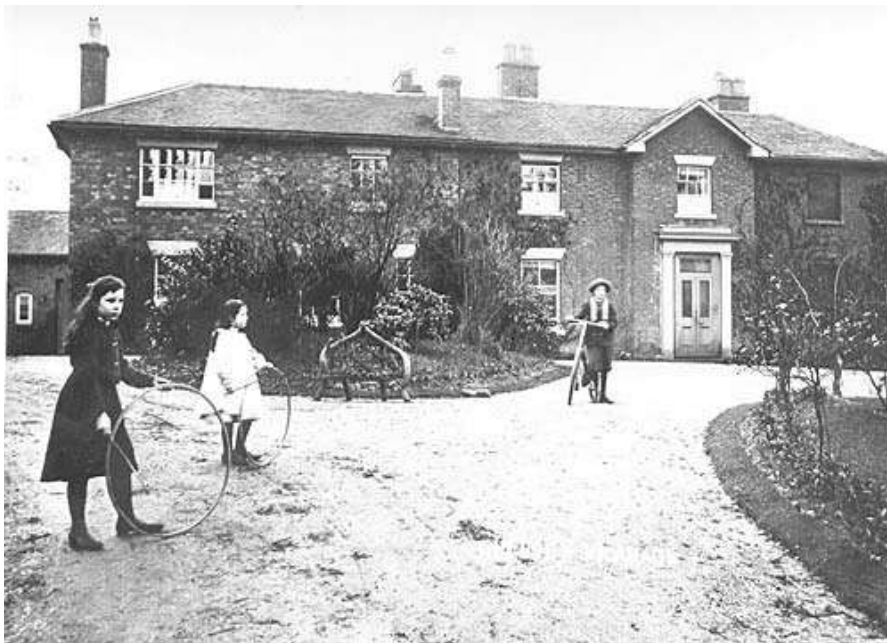
Figure 39 The Old Vicarage in c.1900. Many original features have been retained including some sash windows.
