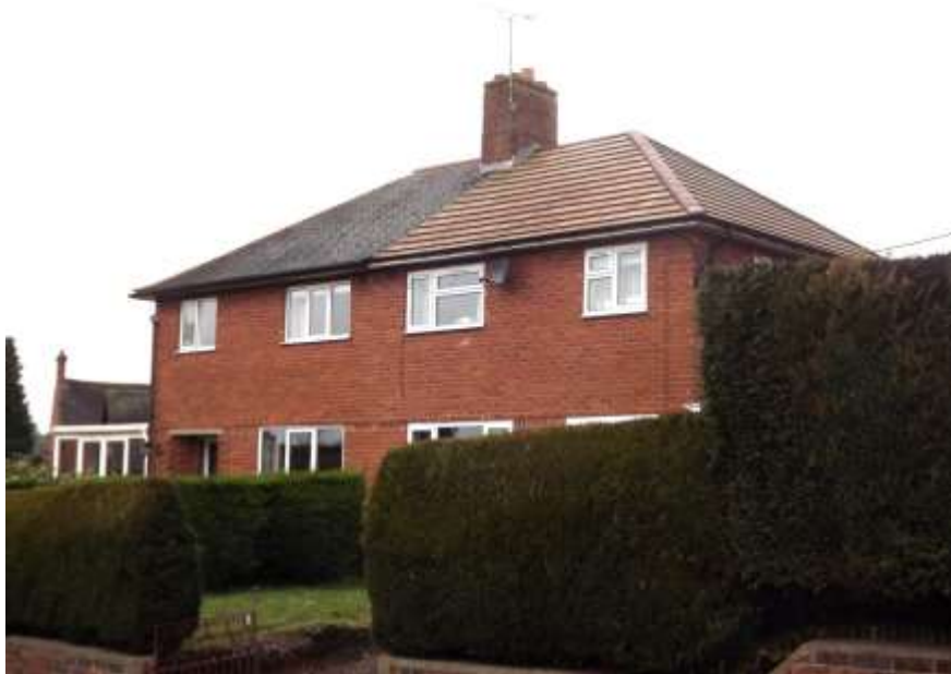
Figure 65 Inappropriate roof tiles create a negative impact
