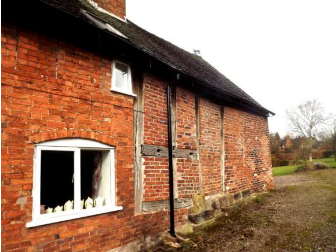
Figure 22 Exposed timber frame to the Old School House
